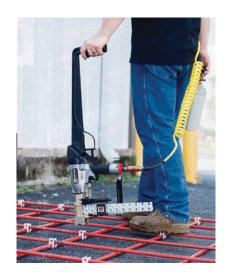
Handle allows a Worker to operate any KLIPPING TOOL from a standing position, eliminating the need to bend, stoop, or crouch while
