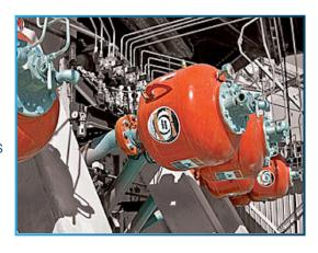
valve that, when strategically located and properly oriented and controlled (automatically or manually), creates an eruptive blast that unclogs, dislodges, and prevents the material build-up that chokes plant productivity and efficiency.
