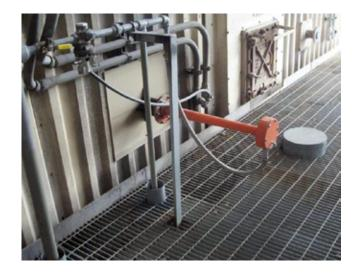
Because Sonic Horns operate at frequencies higher than the resonance frequency of steel, ceramic linings, concrete, etc, they do not cause vibrational damage to the vessel or surrounding structure. Suitable for explosive environments, Sonic Horns have not only been used for vessel cleaning, but also for maintaining air preheaters, precipitators, SCR reactors, heat exchangers, filters, boiler tubes, baghouses, draft fans, and ductwork.
